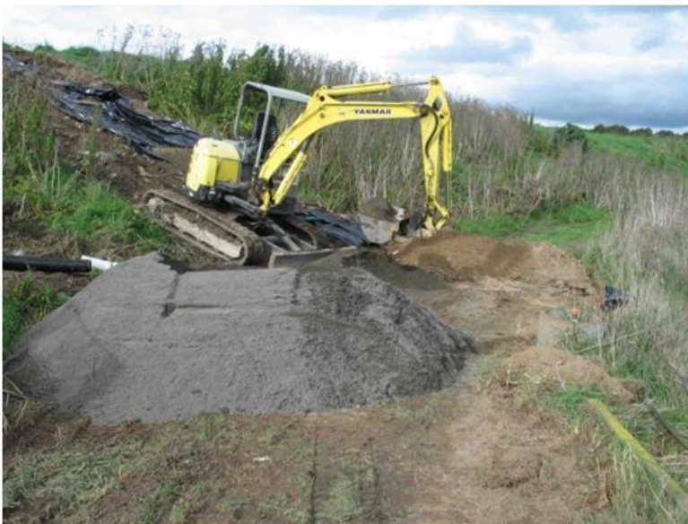
Figure 4 mixing sand and pumice
