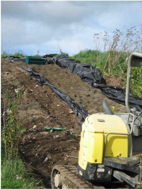
Figure 5 Filling the trench
